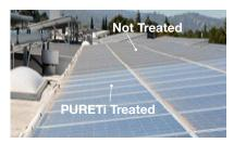
PURETi Clear is a spray applied, water based, light activated, pollution reversing, architectural surface treatment
